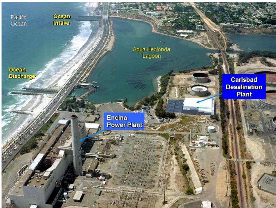
Figure 1 - Carlsbad Seawater Desalination Project
