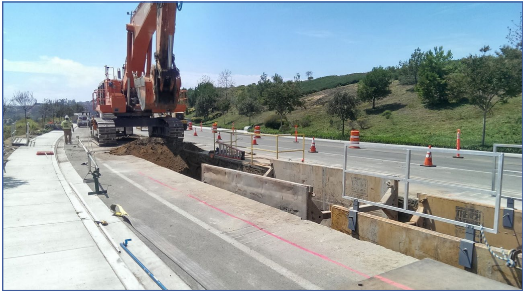
Pipeline installation continues along Faraday Avenue.
