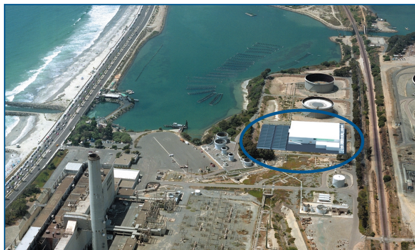
Artist Rendering of Carlsbad Desalination Plant at the Encina Power Station
